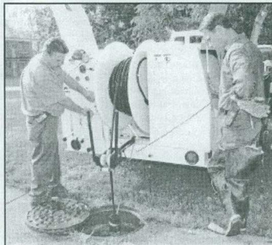
**SUCK IT UP:** Physical plant plumbers Stephen Klein (left) and Terry Schaefer operate the Shamrock Sewer Jetter that is used to clean sanitation and storm water drains on campus. The high-powered machine has saved time and money compared to formerly paying contractors to do the work.
