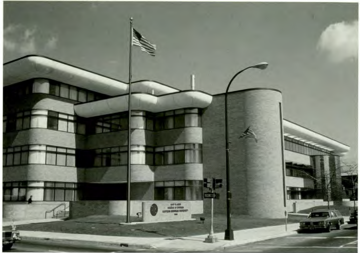
The Gary M. Owen College of Business Building opened in downtown Ypsilanti in 1991.
