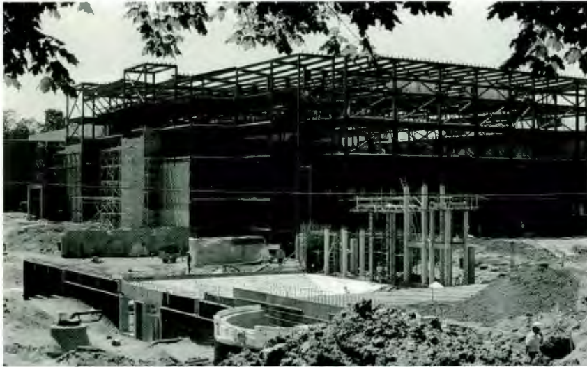
Construction of the intramural facilities, July 1981.
