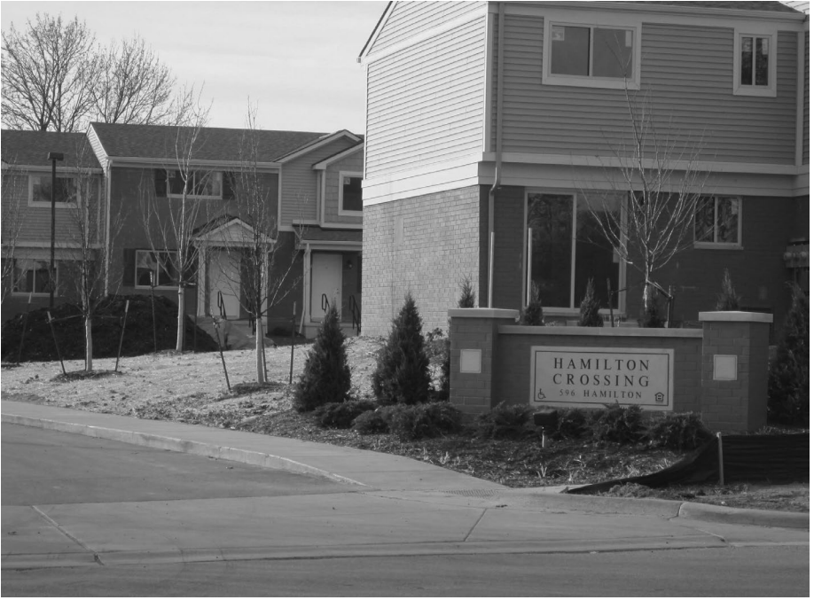
Hamilton Crossing: the finished product
