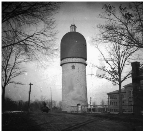
The most noted landmark in the city of Ypsilanti, the Water Tower was erected as part of the city water system, of which it is still a part
